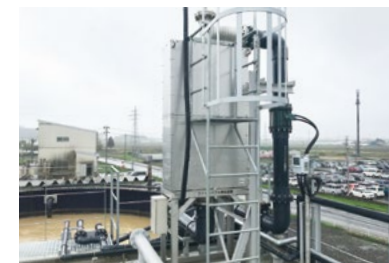
The foam jet system is a highly efficient aeration system that supplies oxygen in fine bubbles. Various benefits can be achieved by diffusing fine bubbles into wastewater.
